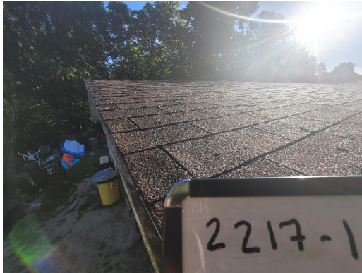
2217-1 Asphalt Shingle/Tar Typical Exterior Roof
