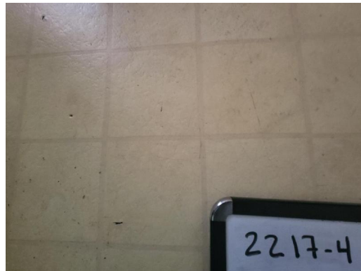
2217-4 Rolled Flooring/Mastic Interior Kitchen
