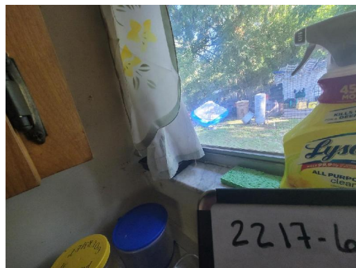
2217-6 Caulk Typical Interior Windows
